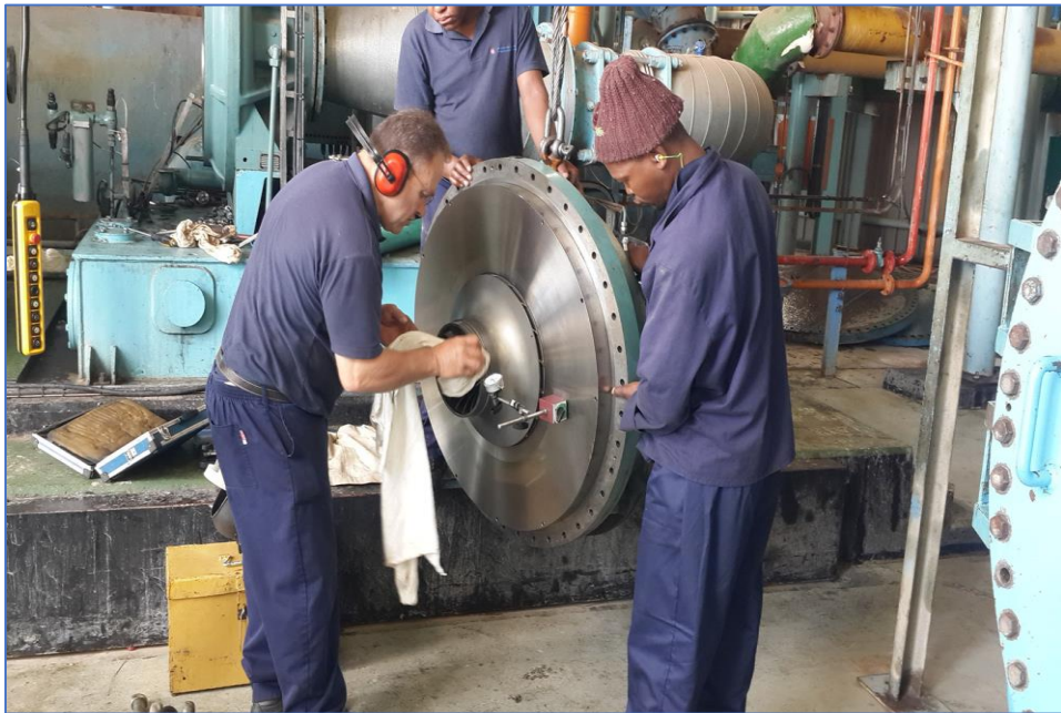
York YK J4 Compressor Float inspection
