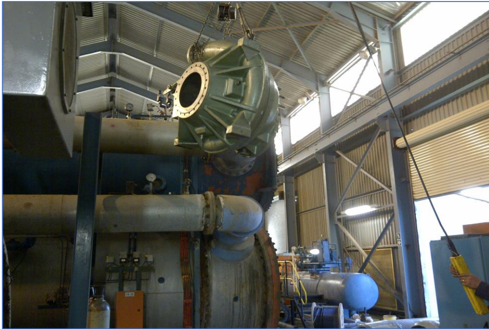
Removal of York YK J4 Compressor
