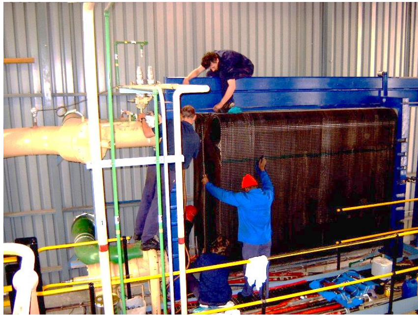
Ammonia Plate heat exchanger
