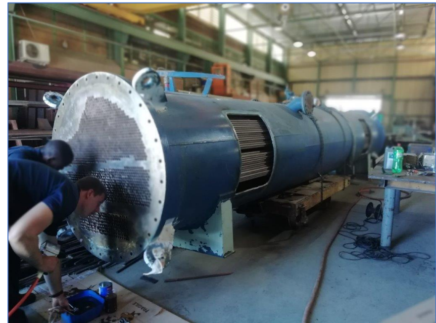
Condenser tube expansion as per OEM specification
