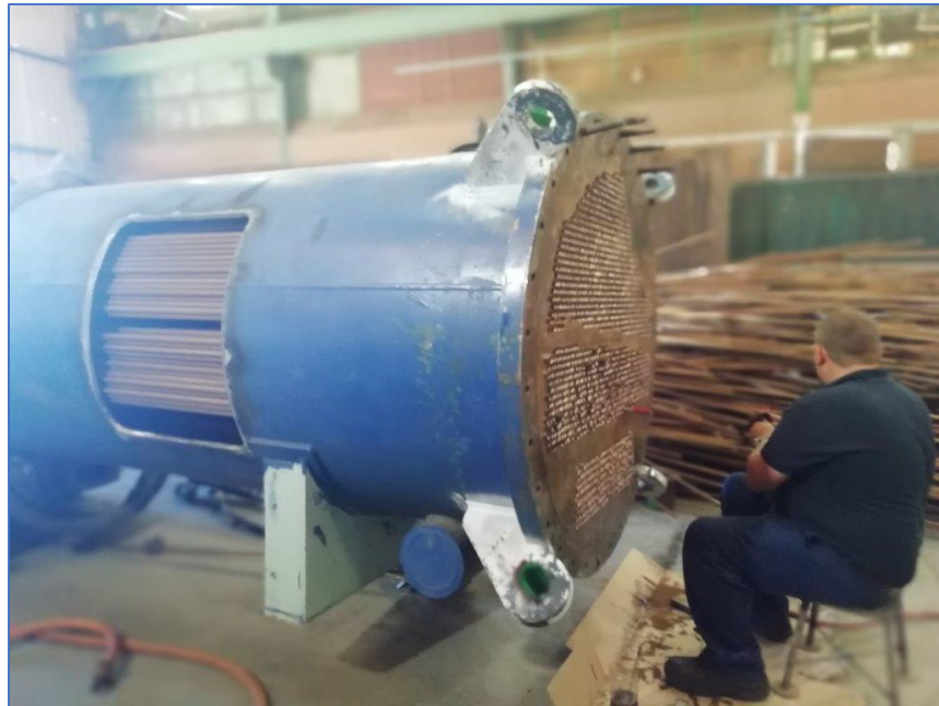
Condenser tube replacement
